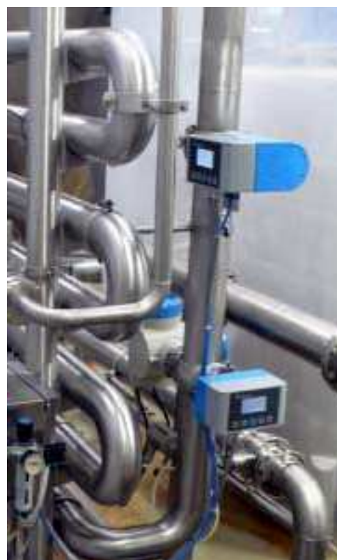
Centec In-Line Process measurement for Original Gravity, Alcohol, Oxygen and carbon dioxide
